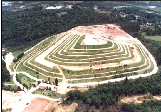
Gambar 9: Penataan TPA Sanitary Land-fill
